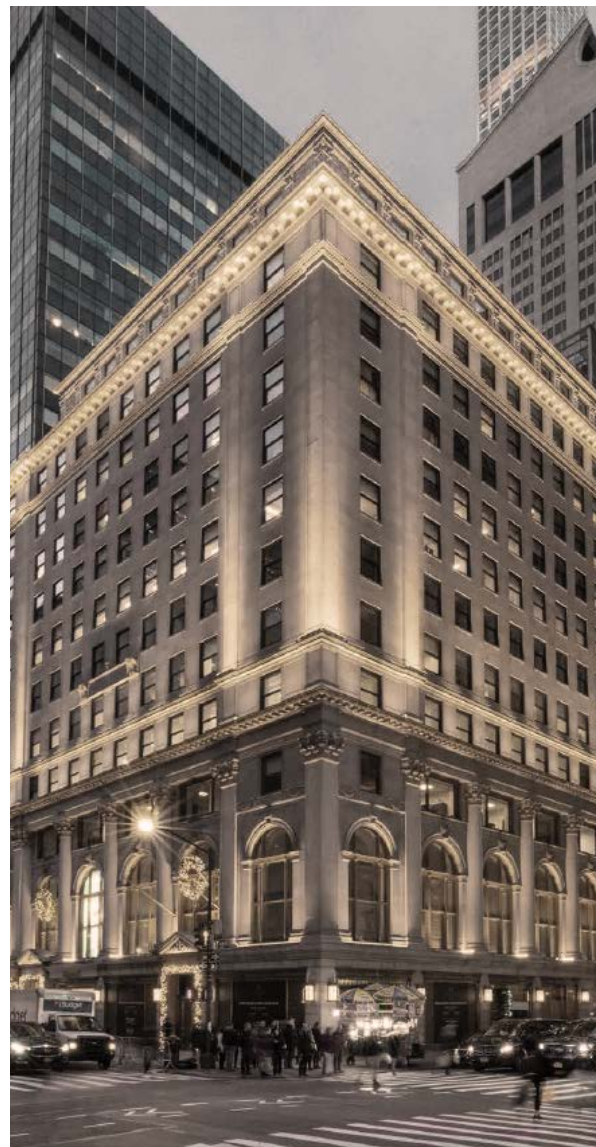
COCA COLA BUILDING 711 FIFTH AVENUE - NEW YORK ▼
